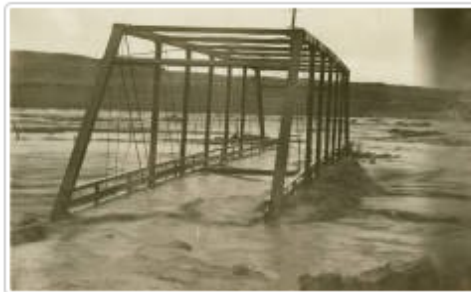
1910 Flood at Hooper WA (WRH Image)
