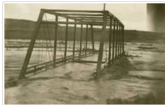
1910 Flood at Hooper WA (WRH Image)
